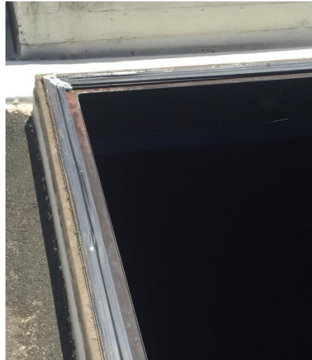
Ventilation unit rubber seals
